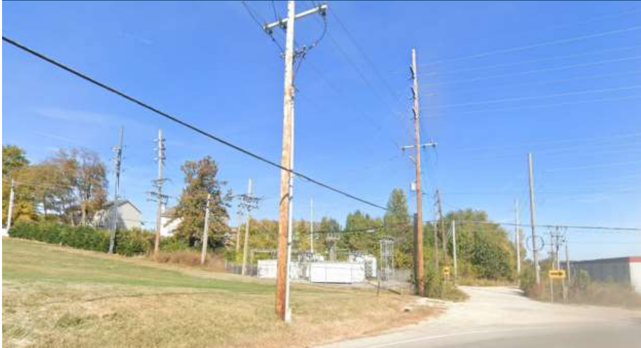
FIGURE 4: GOOGLE STREETVIEW OF SUBSTATION AND INFRASTRUCTURE, OCT. 2022
