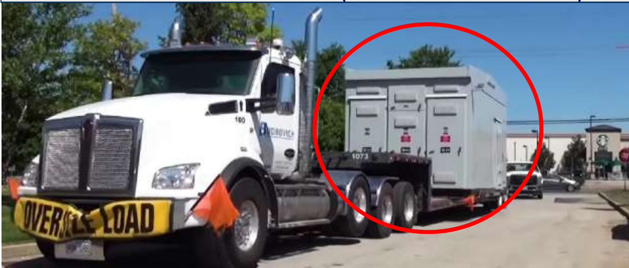
FIGURE 2: EXAMPLE OF SWITCHGEAR STRUCTURE (PHOTO: AMEREN MO MARKETING)
