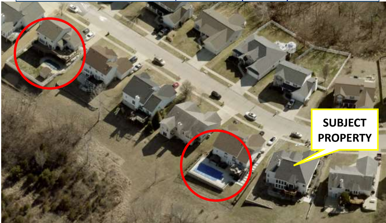
FIGURE 4: PICTOMETRY OF SUBJECT SITE, FACING SOUTH (MAR. 2022)
