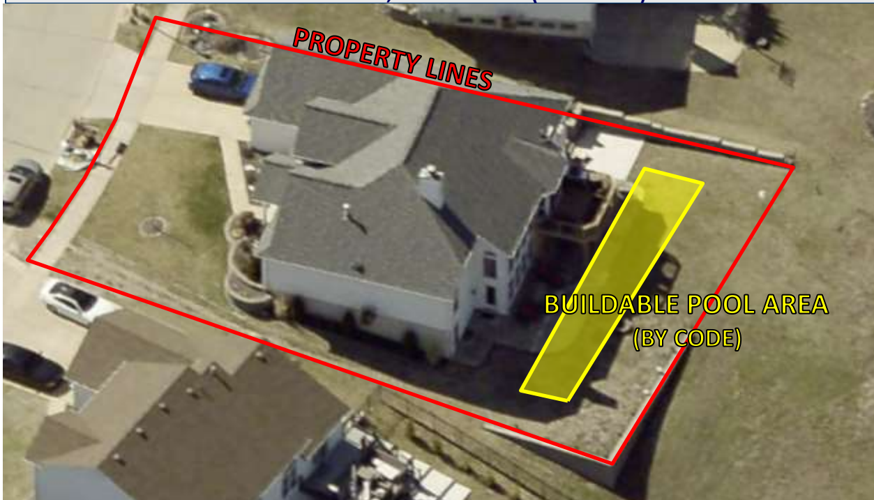
FIGURE 5: PICTOMETRY OF SUBJECT SITE, FACING WEST (MAR. 2022)
