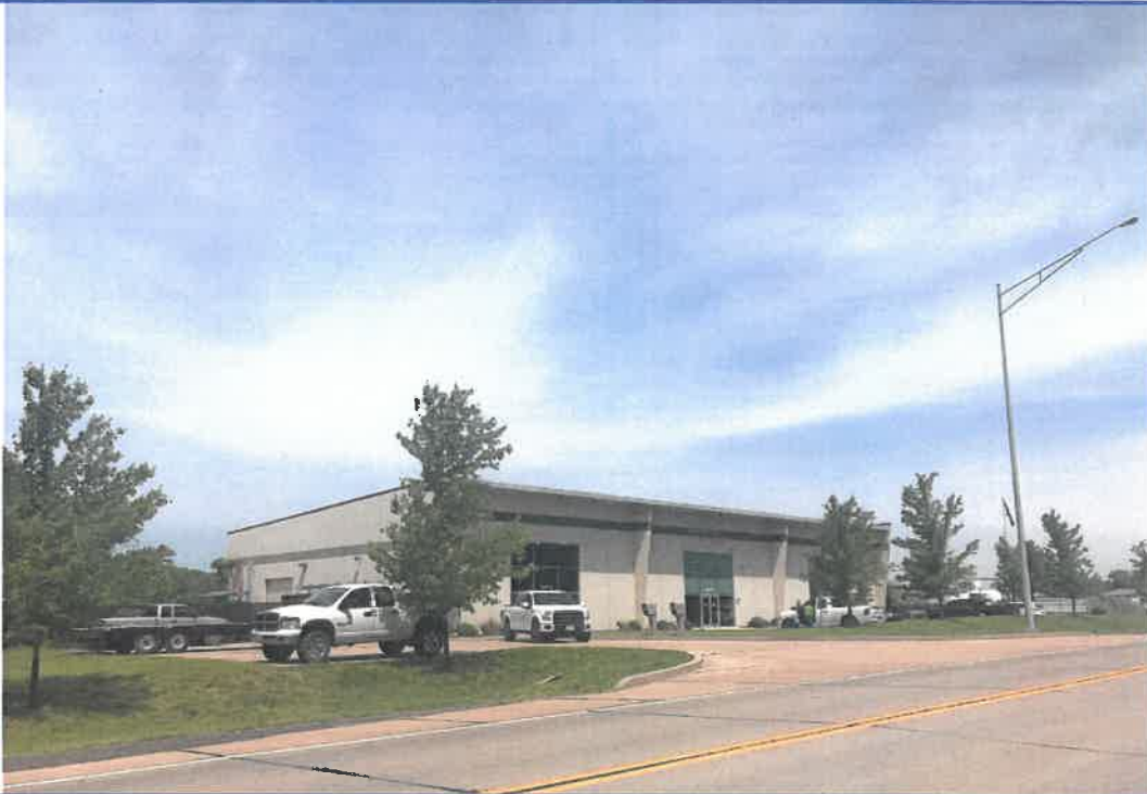
PUBLIC VIEWSHED OF SPENCER CONTRACTING FROM ARNOLD TENBROOK FACING NORTHWEST
