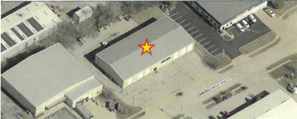
FIGURE 3: CURRENT LOCATION OF CAPE ELECTRICAL SUPPLY (PICTOMETRY, MARCH 2022)
