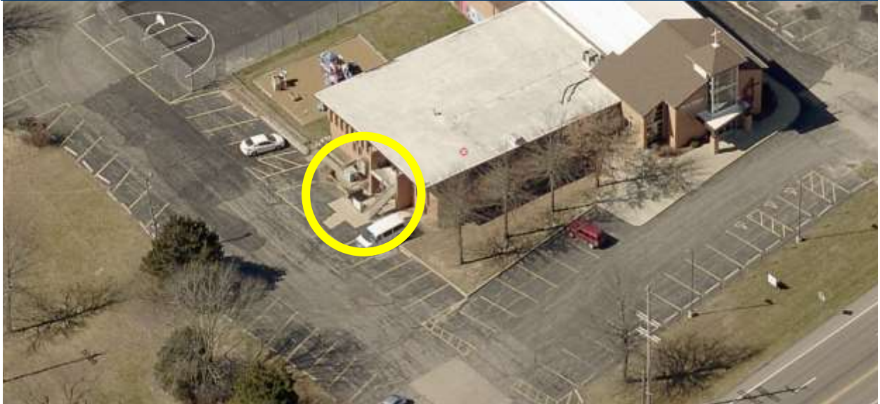
FIGURE 2: VIEW OF NEW HOPE UMC FACING EAST; HEAD START ENTRANCE CIRCLED IN YELLOW
