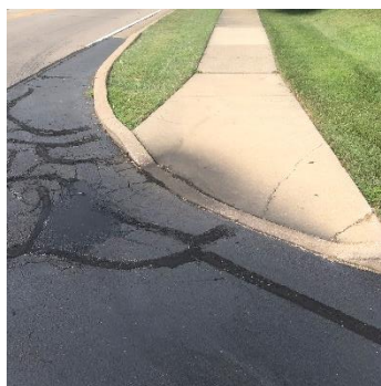
_____ No Detectable Warning Panels (e.g. bumps at the bottom of the curb ramp)
